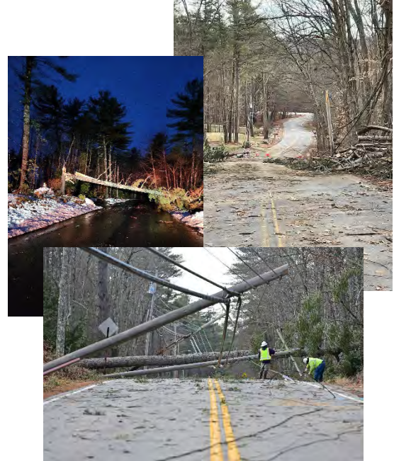
Figure 1 - Storm Damage NH
